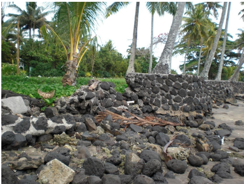
Figure 12: Damaged Coastal Defences in Independent Samoa
