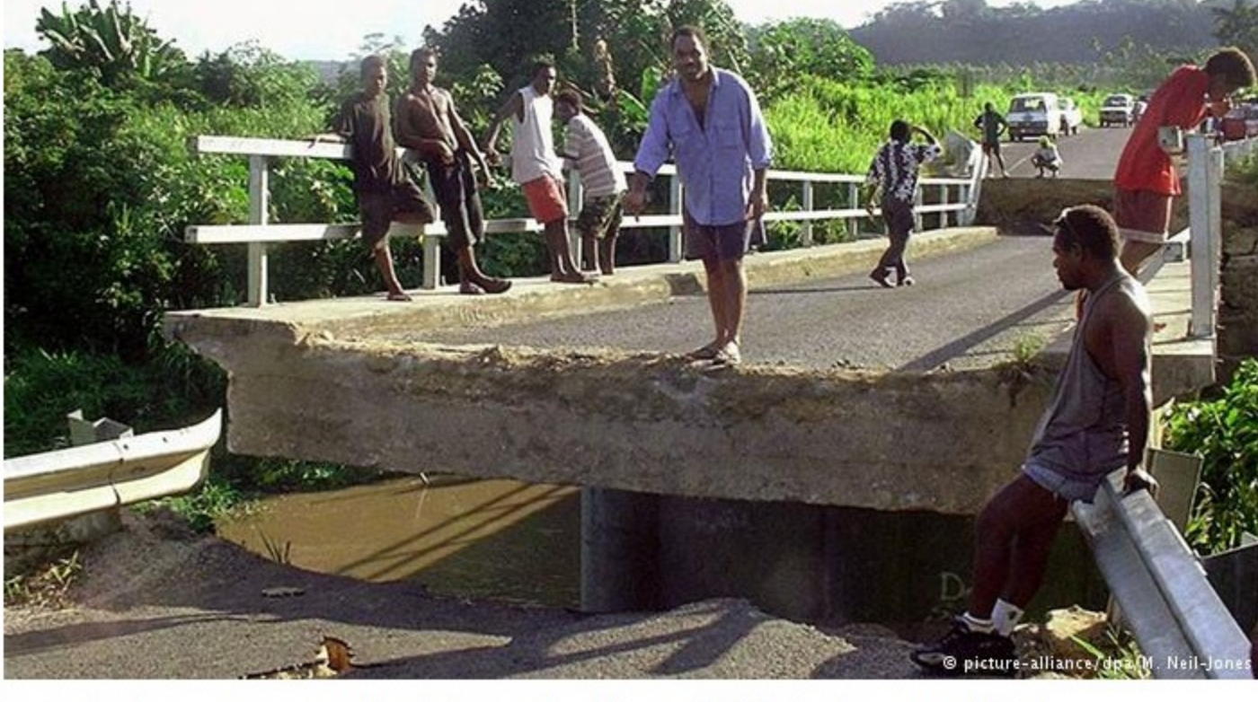
Destruction from a 7.4 Vanuatu earthquake in 2002 for which no official death toll was ever published
