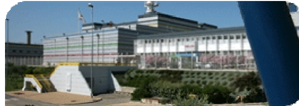
MELOX - MOX fuel fabrication plant
