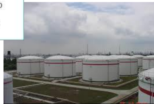
Oil Tank : 0.02 €/kWh
