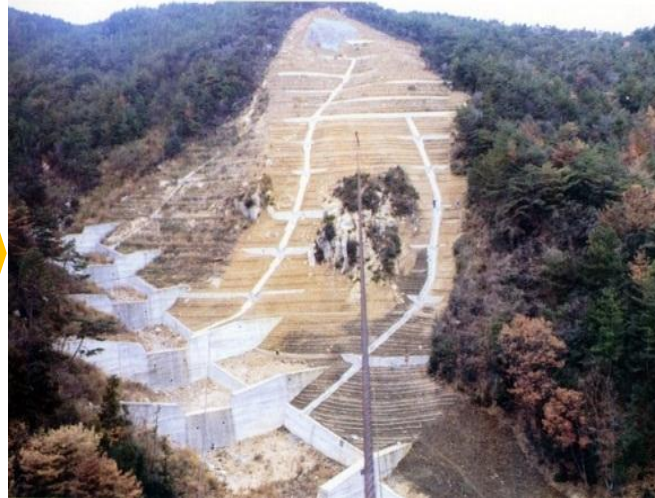
Under the work
