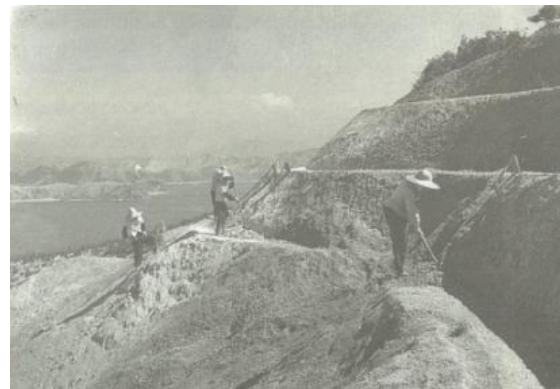
Under the work (Stair Slope Work) (around 1953)
