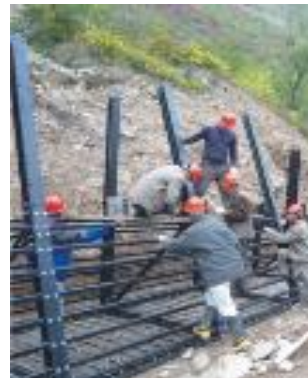
Under the work
