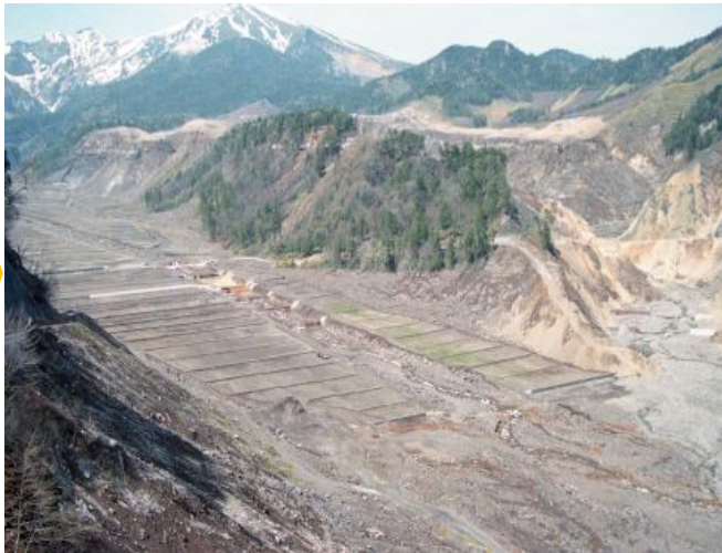
Under the work
