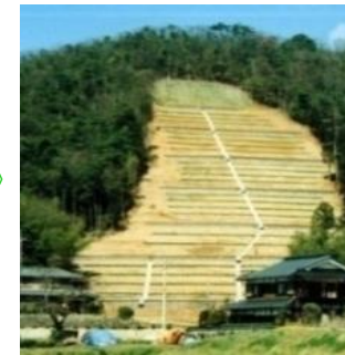
Immediately after the work (1998)
