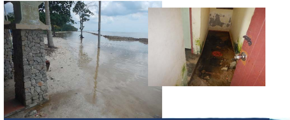
Punggur Recreational Park is impacted by sea water - saline intrusion extends to almost 10 m inland.
